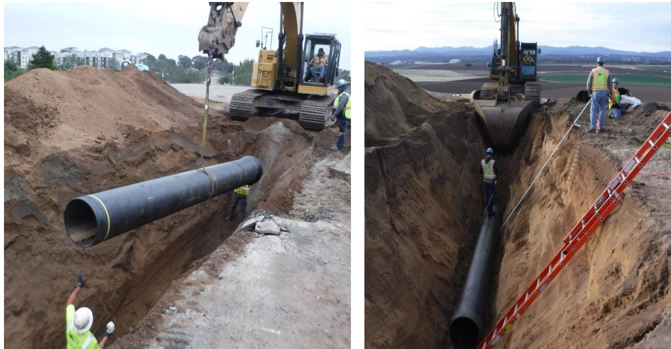
Construction of the MCWD's RUWAP Transmission Pipeline that will serve both MCWD customers and M1W's Pure Water Monterey Project which was recently completed.
