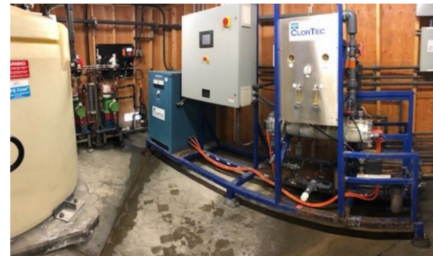
Old Chlorine Generator
